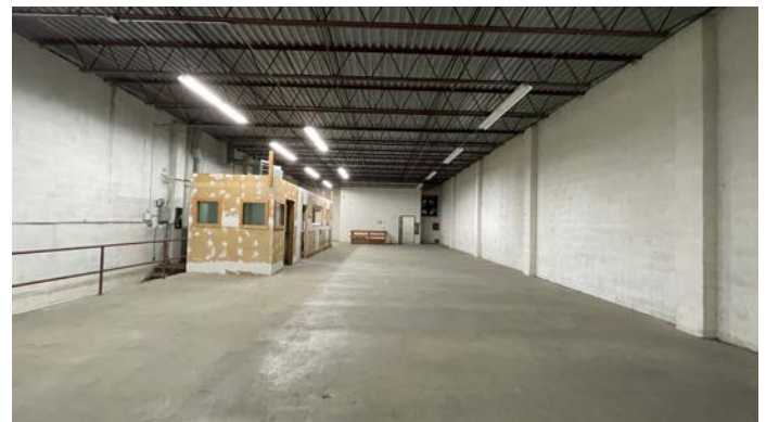
CLEAR SPAN CONSTRUCTION
