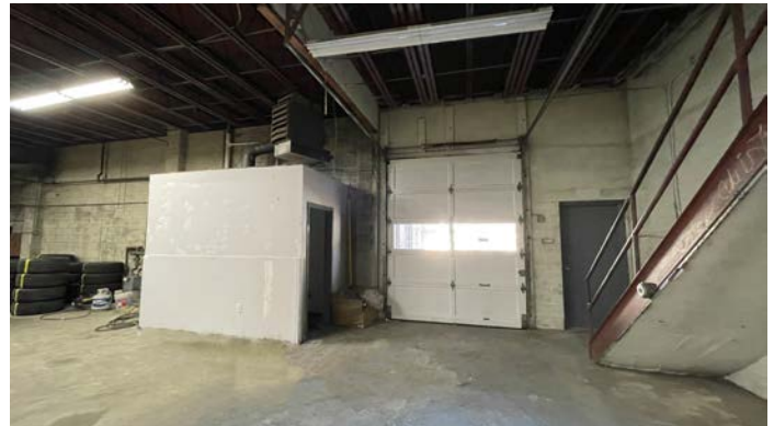
OVERHEAD DOOR ACCESS TO COVERED DOCK
